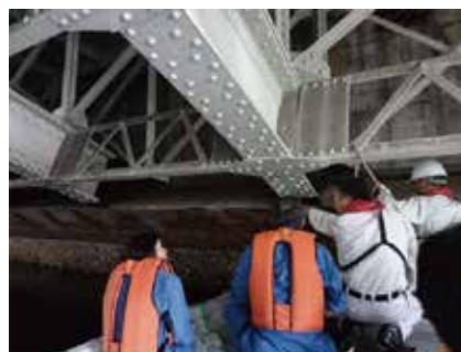
Checking of Beam
