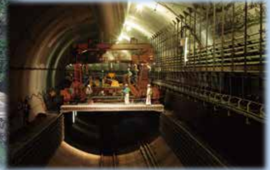
Ring Expressway North Line at Underground Section (under construction)
