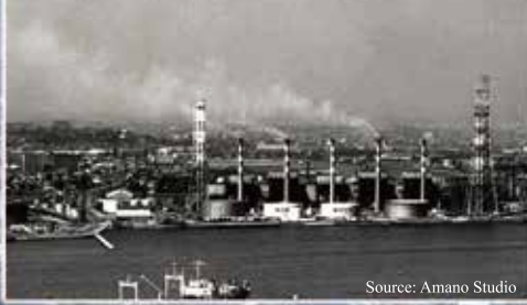
Industrial Zone of Yokohama Bay Area (Past)
