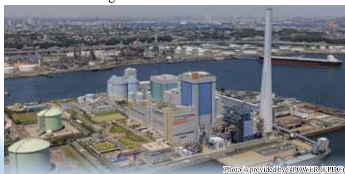
Isogo Thermal Power Plant
