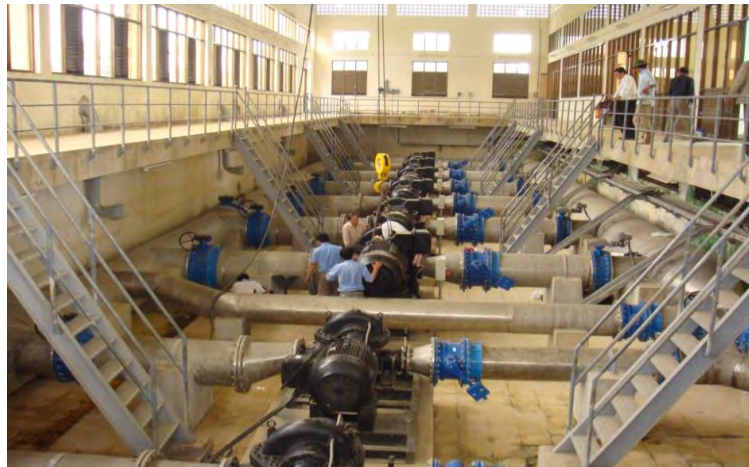
Applying JCM model to installation of high efficiency pumps at DAWACO (2016)
