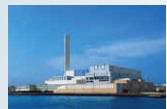
Kanazawa Incineration plant
