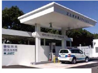
Kitakyushu hydrogen station
